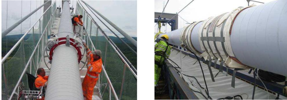
Figure 9 Wrapping with wrapping machine and bonding with heat blankets
