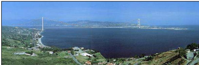
Figure 7 The Messina Bridge, Italy – world record span of 3,300 m
