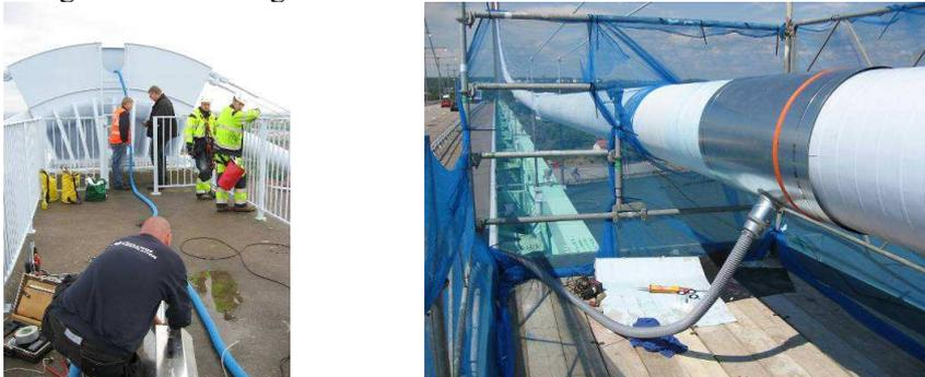
Figure 14 Injection and flow testing at tower saddle and mid span on the Älvsborg Bridge, Sweden
