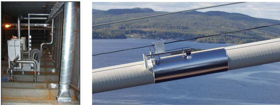
Figure 8 Dehumidification plant and exhaust sleeve
