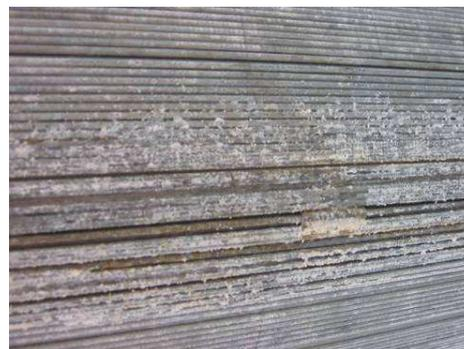
Figure 1 Corrosion on main cables aged roughly 30 and 8 years
