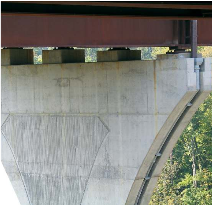
Cover Bridge Photo: Veterans Memorial Bridge, Portland, ME - Versiflex™ HLMR Disc Bearing Assemblies by The D.S. Brown Company.
