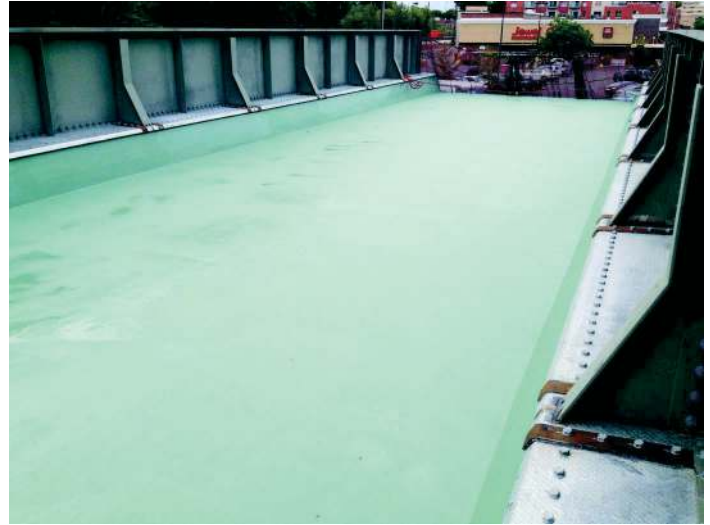
Deckguard® Waterproofing System, Greenleaf Avenue Bridge, Chicago, IL
