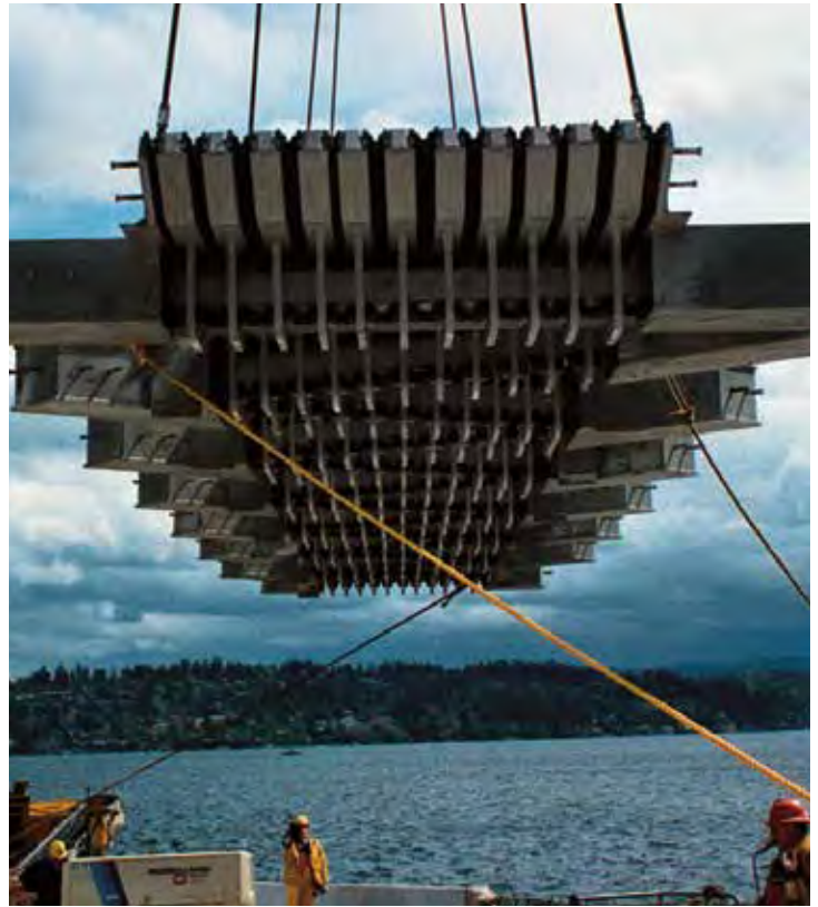
Lacey V. Murrow Floating Bridge, Seattle, WA, USA
