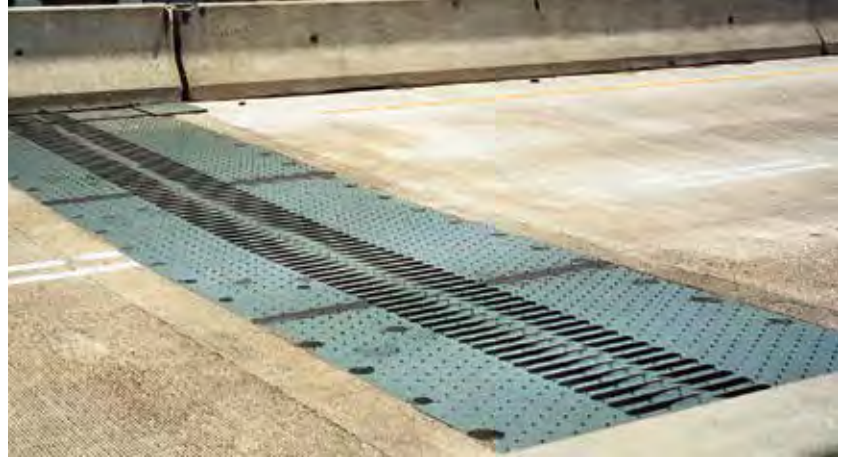
Finger Joint Assembly
