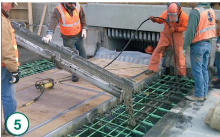
The following is a recommended procedure for the installation of swivel expansion joints. Consult contract plans and D.S. Brown shop drawings for blockout dimensions, placement of the joint, and the effects of temperature on their positioning.
