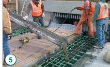
The following is a recommended procedure for the installation of swivel expansion joints. Consult contract plans and D.S. Brown shop drawings for blockout dimensions, placement of the joint, and the effects of temperature on their positioning.
