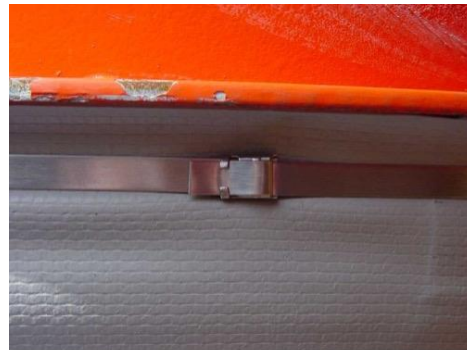
FIGURE 23: STRAP INSTALLED BEHIND INDICATOR BUMP
