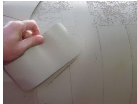
FIGURE 36: PATCH 100 mm LONGER THAN CUT
