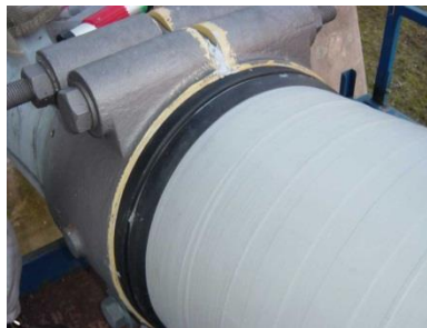
FIGURE 8: WEDGE INSTALLATION
