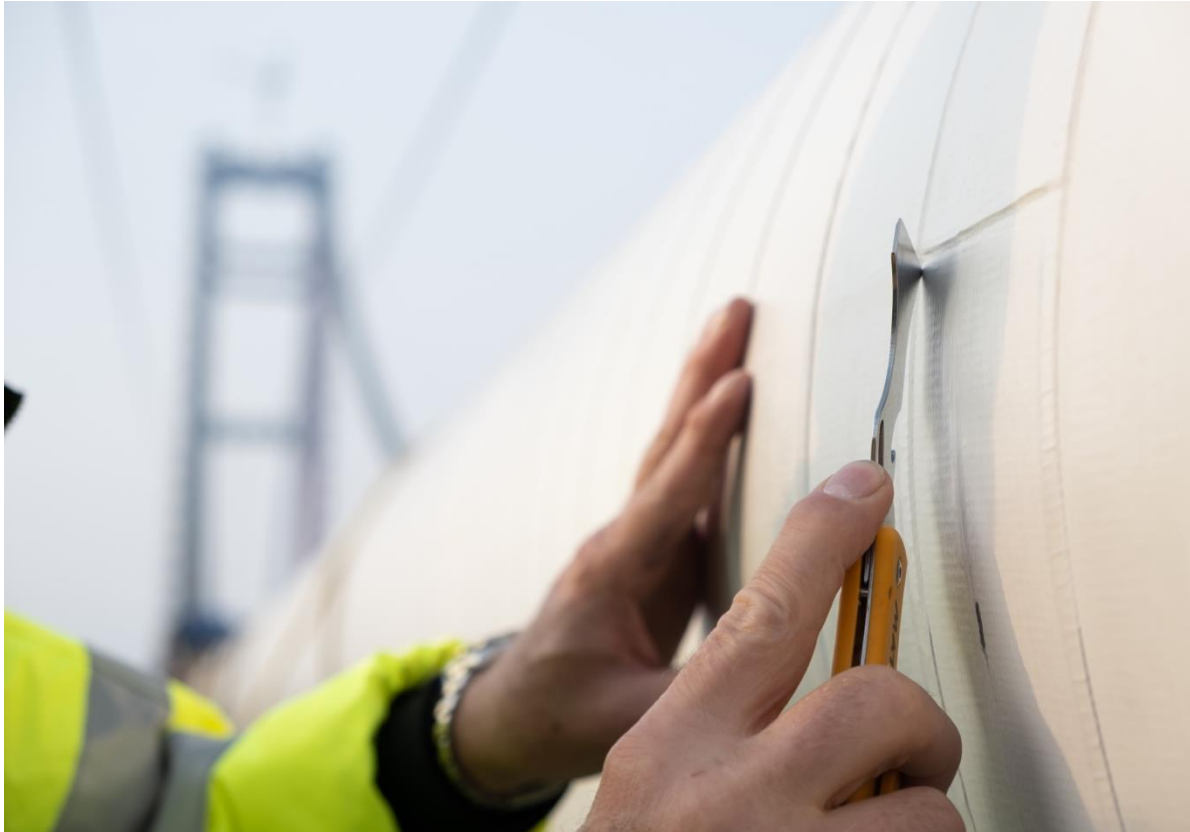
FIGURE 6: SEAM TESTING FOR ACCEPTABLE BOND
