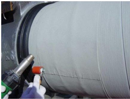
FIGURE 20: HEATING FINISH STRIP
