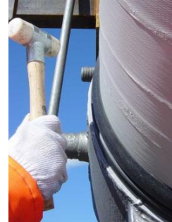
FIGURE 15: SLIDING WEDGE INTO PLACE
