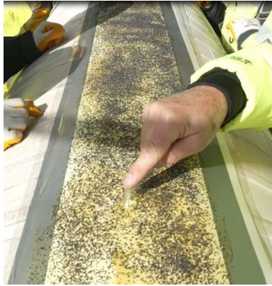
FIGURE 29: BASE COAT LIFTING AND NOT READY FOR TOP COAT APPLICATION
