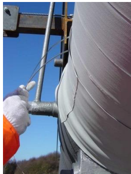
FIGURE 22: FINISHED STRIP SNAPPED OVER WEDGE
