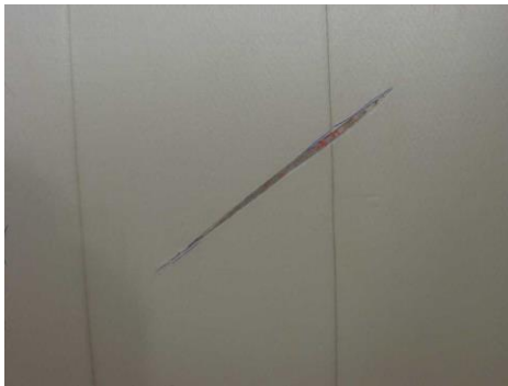
FIGURE 35: CUT LESS THAN 75 mm LONG
