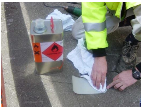
FIGURE 37: CLEAN PATCH WITH XYLENE
