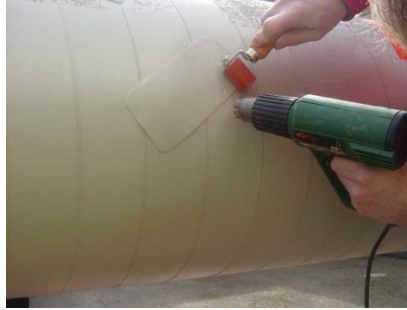
FIGURE 39: APPLY THE PATCH USING A HEAT GUN AND ROLLER
