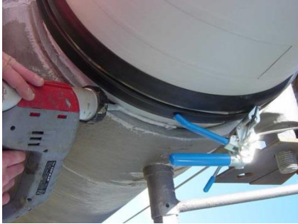
FIGURE 14: APPLYING SEALANT
