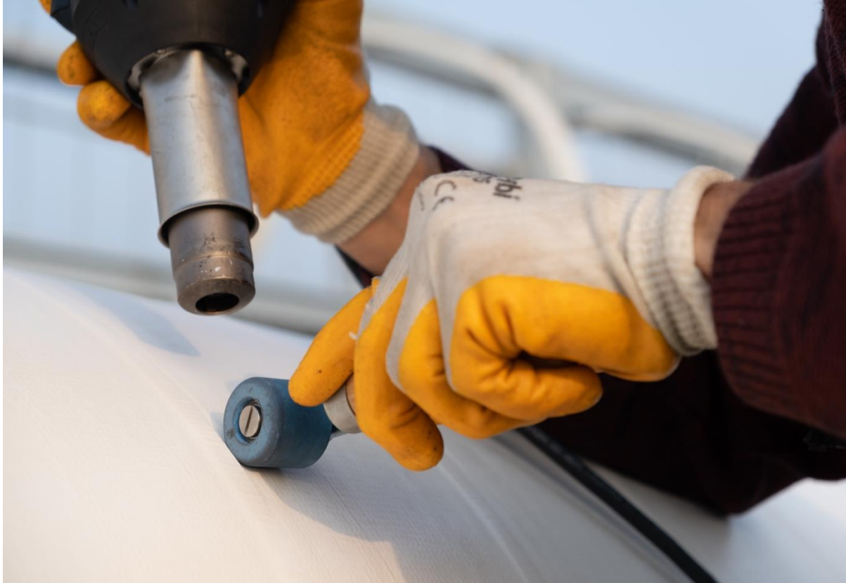
FIGURE 7: EDGE SEAMING WITH A HEAT GUN AND HAND ROLLER
