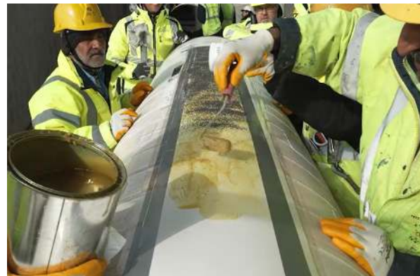
FIGURE 28: BASE COAT AND GRIT APPLICATION
