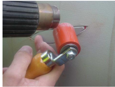
FIGURE 43: APPLY FILLER PATCH WITH A HEAT GUN AND ROLLER
