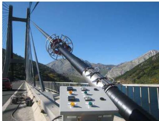
FIGURE 34: CABLESTAY INSTALLATION WITH CLAMSHELL STYLE HEATER
