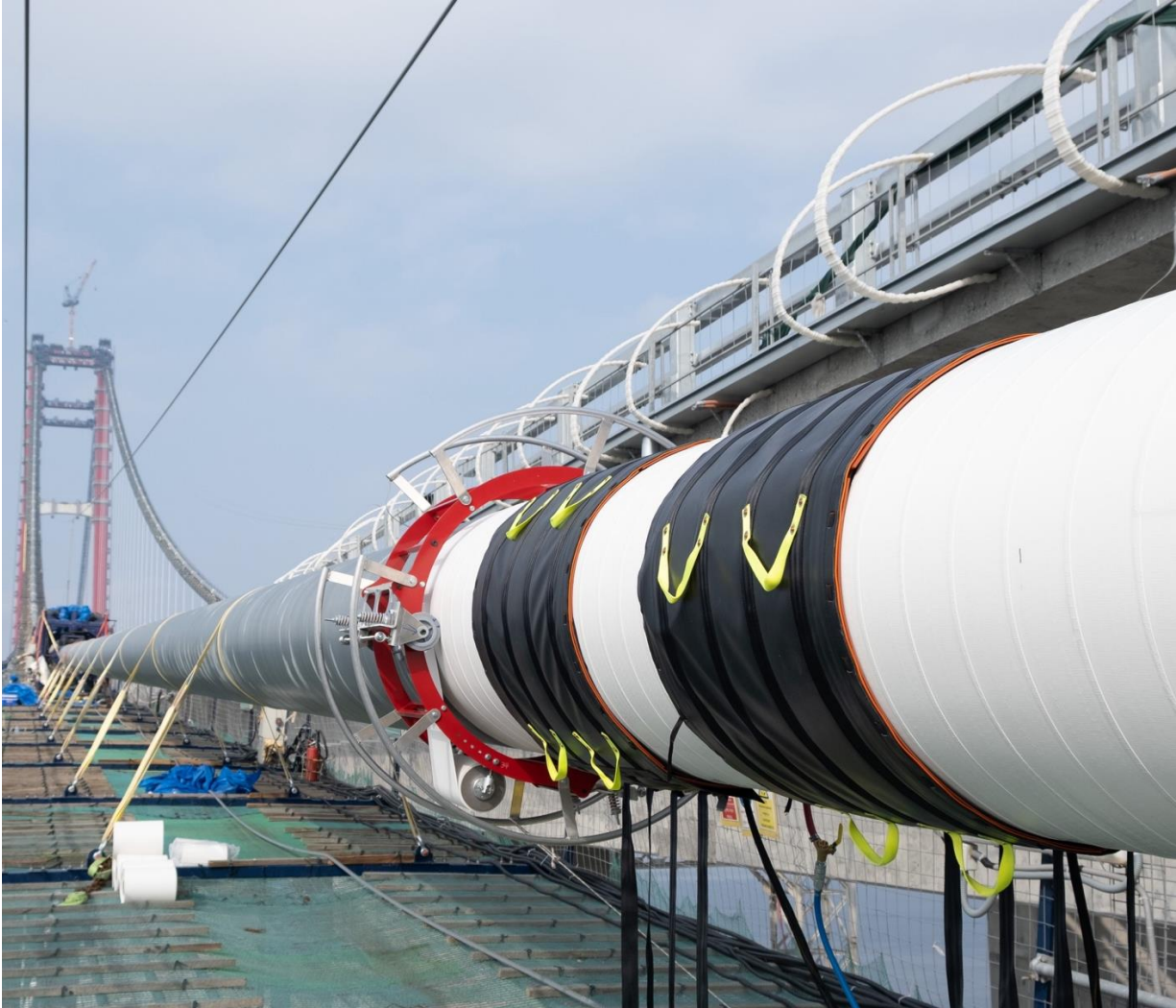
Cableguard™ Elastomeric Wrap System installation on the 1915 Çanakkale Bridge spanning the Dardanelles Strait, Turkey
