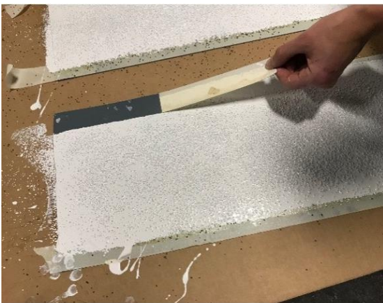
FIGURE 31: MASKING TAPE BEING REMOVED IMMEDIATELY AFTER TOP COAT APPLICATION
