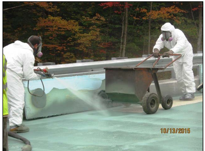
Deckguard sprayed on surface ahead of aggregate broadcast with a spreader/seeder.
