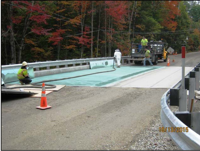
The spray-applied membrane application was performed by Sealcoating, Inc. from Braintree, MA
