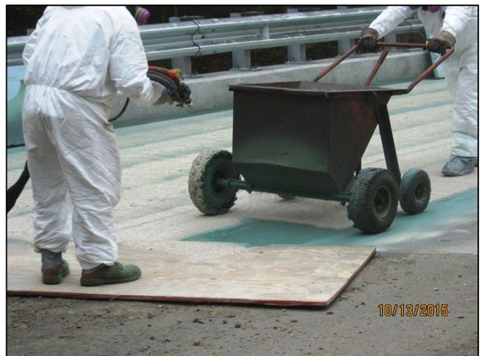
Application of a second 20 to 30 mil layer of membrane along with an aggregate broadcast for shear-key purposes.
