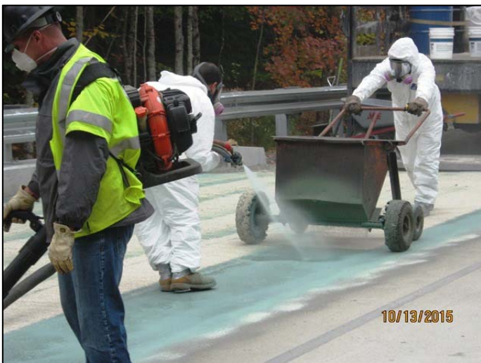
Application of a second 20 to 30 mil layer of membrane along with an aggregate broadcast for shear-key purposes.
