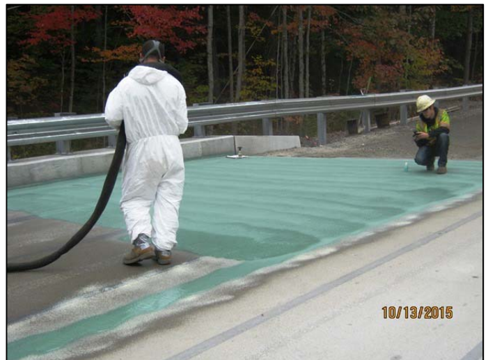
Quality assurance tests (pull-off) were performed throughout the application process.
