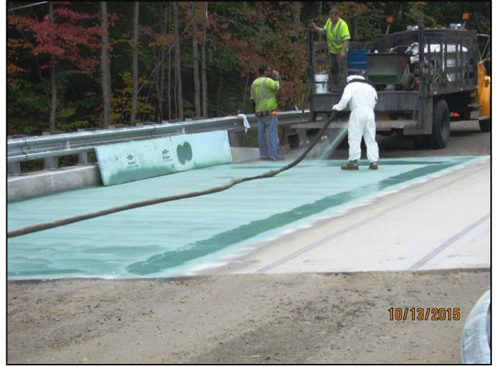
The spray-applied membrane application was performed by Sealcoating, Inc. from Braintree, MA
