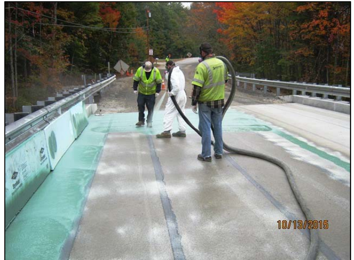
Deckguard Spray Membrane is applied over the Deckguard Primer at a nominal 80 mil thickness.
