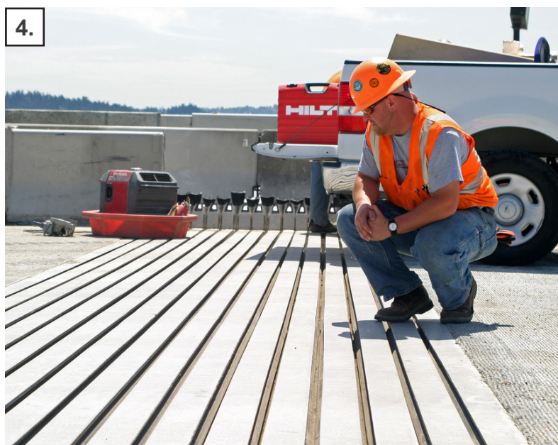
2. WSDOT project engineers and bridge inspectors inspecting an expansion joint upon arrival in Seattle.
