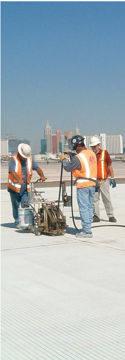
Delastic® Preformed Pavement Seal installation at McCarran International Airport Las Vegas, Nevada
