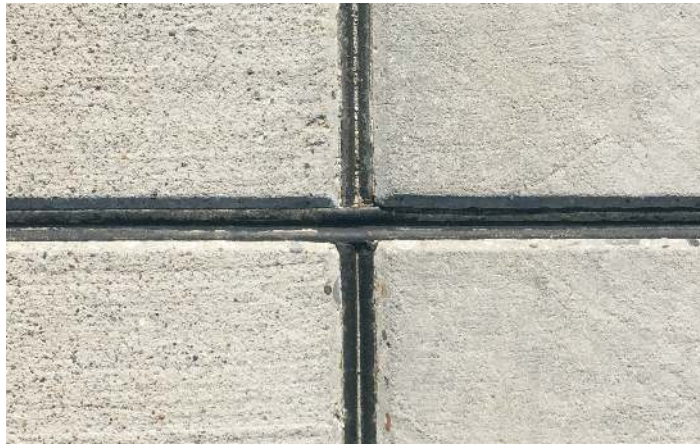
Delastic® Preformed Pavement seals effectively protect concrete pavement in highways, airport aprons and airport runways by keeping moisture, debris and incompressible material out of the joint opening.
