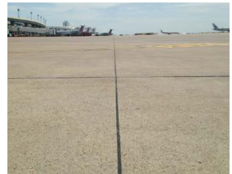
40-year-old Preformed Compression Seal at DFW Airport.
