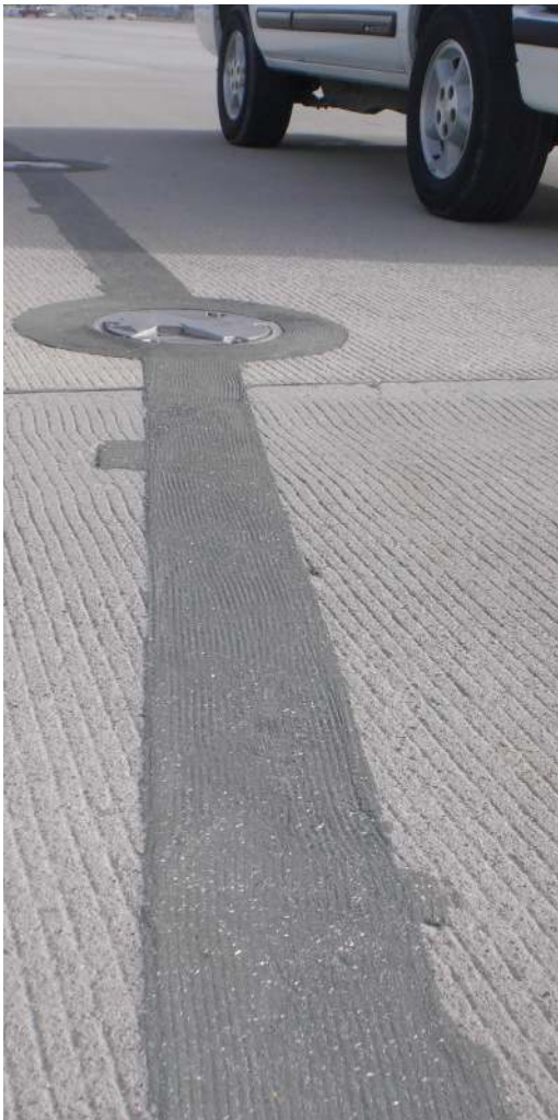
Delpatch™ lighting application, Salt Lake City International Airport, Utah
