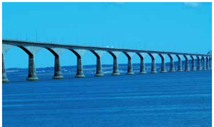
Confederation Bridge, Prince Edward Island, Canada
