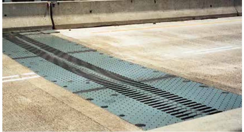
Finger Joint Assembly
