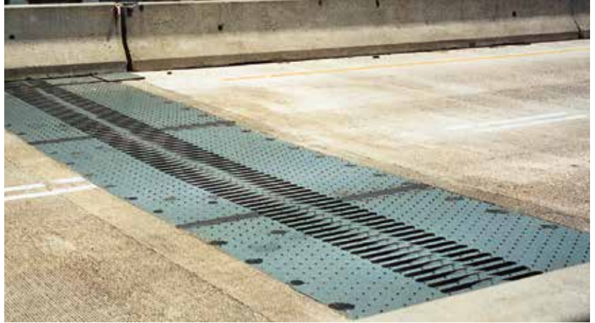
Finger Joint Assembly
