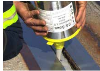
Delastic-LS® Installation
