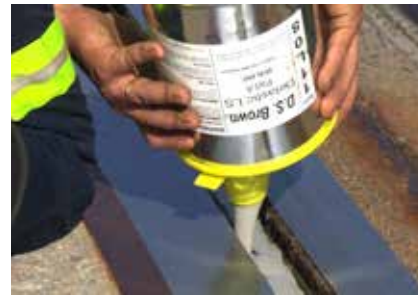
Delastic-LS® Installation
